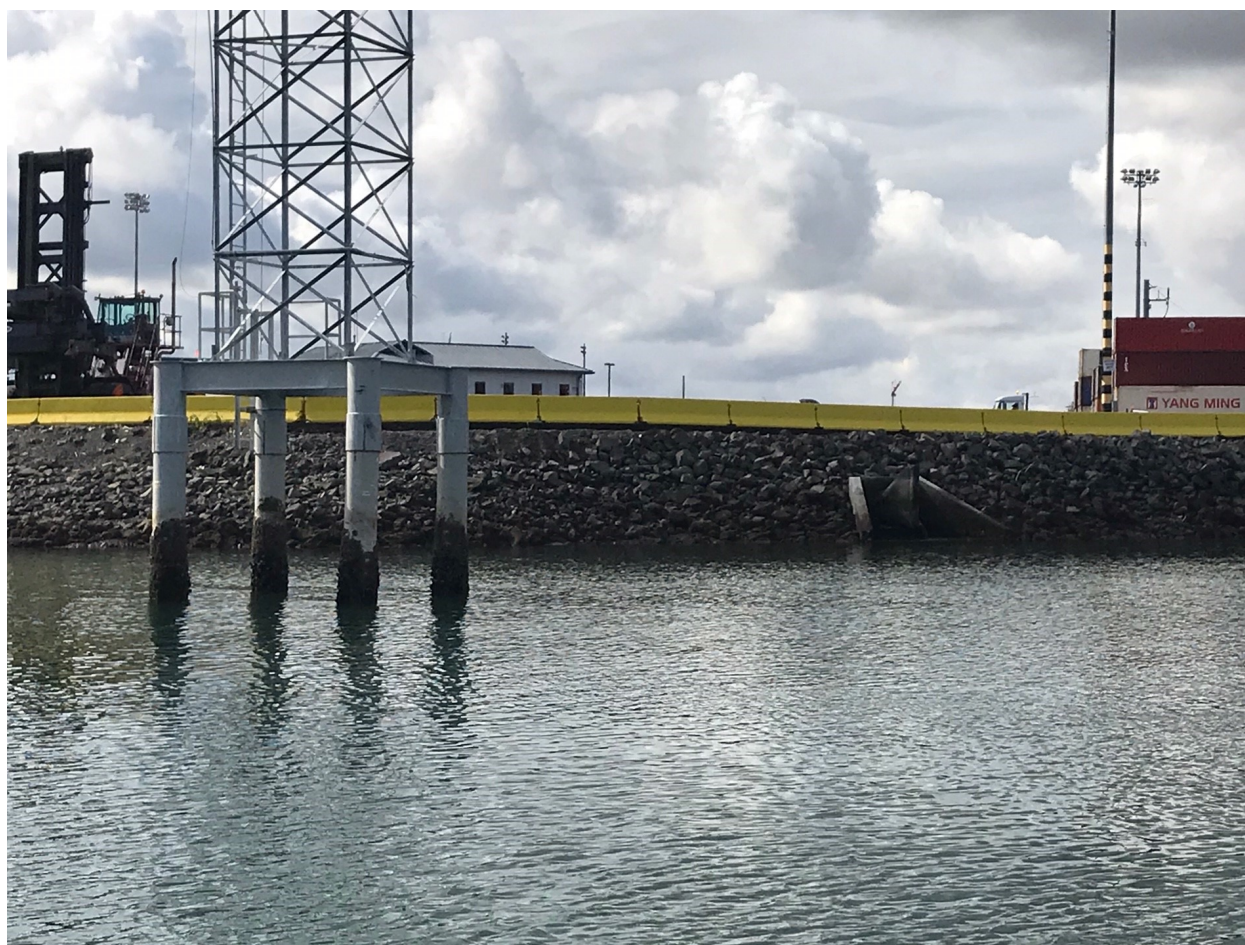
Figure 2: Rip rap shoreline with decommissioned outfall
