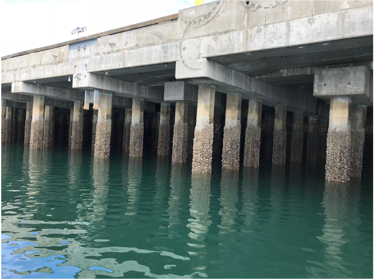
Figure 3: Concrete pilings
